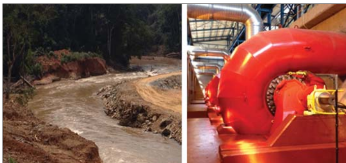
River being prepared for hydropower station and hydro turbine at plant
